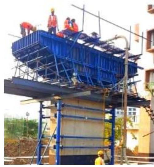
Pier Cap Formwork
